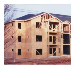
Additionally, panels have a coarse-textured surface with skid-resistant feature that prevents accidents (while working on roofs) and provides an extended adherence area (walls and floors).
